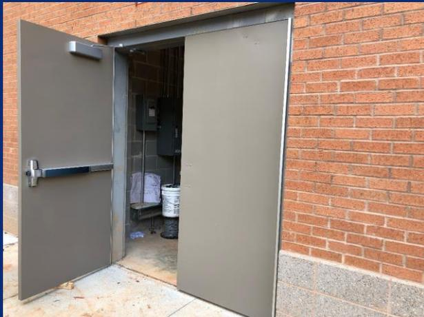
Exterior hollow metal doors installed
