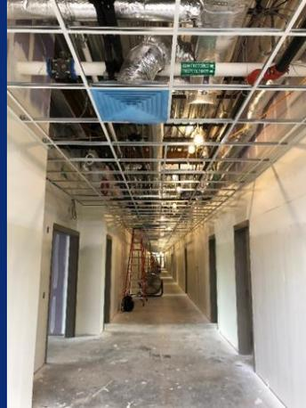
Grid installed and air distribution in progress on 3<sup>rd</sup> level
